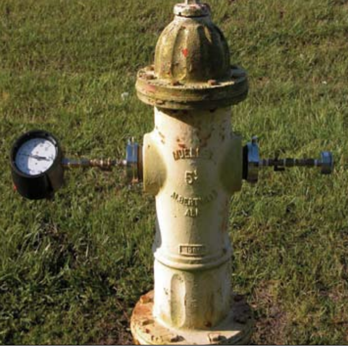
Figure 1. Hydrants were equipped with an analog pressure gauge (left) and a continuous recording pressure (digital) logger (right).
