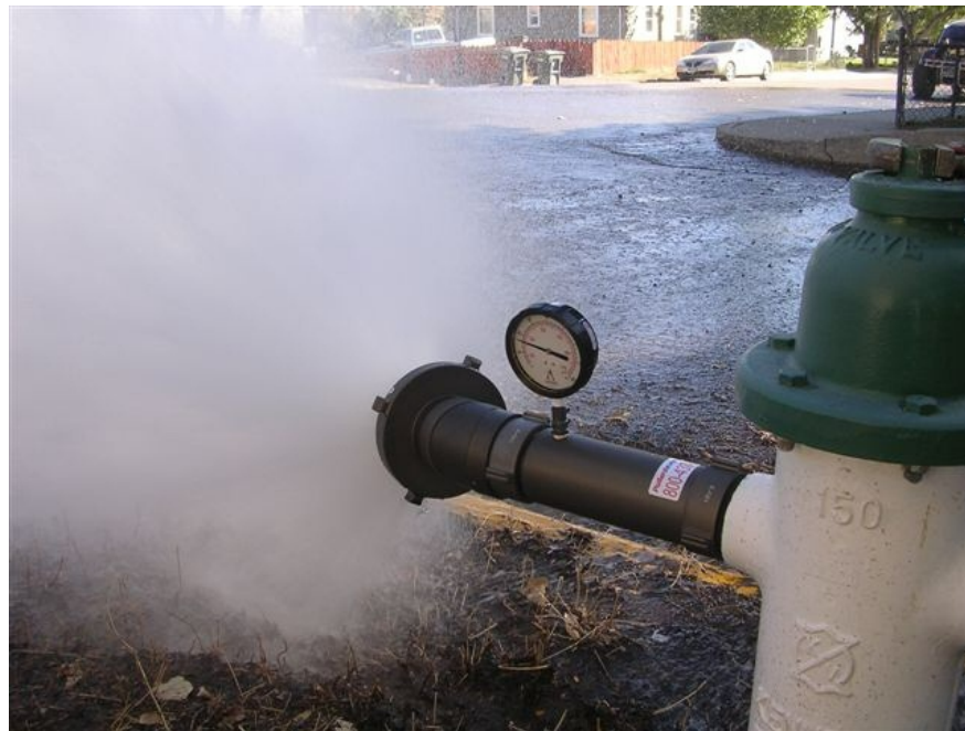
Figure 2. Flow measurement during a hydrant flow test
